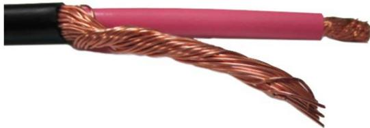
3) Cut the non-insulated copper wire according to RRU requirement.
