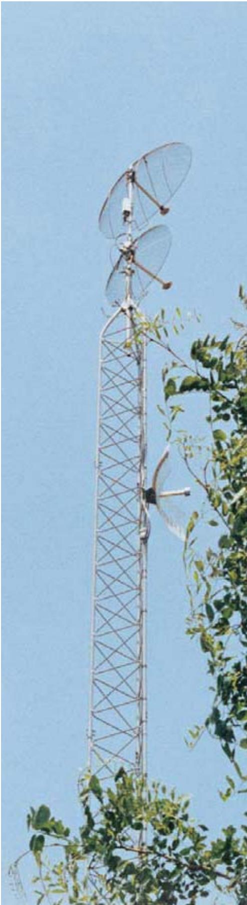
Because of its rugged design, the 55G lends itself to a wide variety of used in the communications field, particularly where unusual wind loading and height requirements exist. The 55G was designed to provide excellent strength in heights up to 400 feet. When properly installed, the standard tower will support loads as shown on various guyed and self-supporting information sheets in the ROHN catalog.
